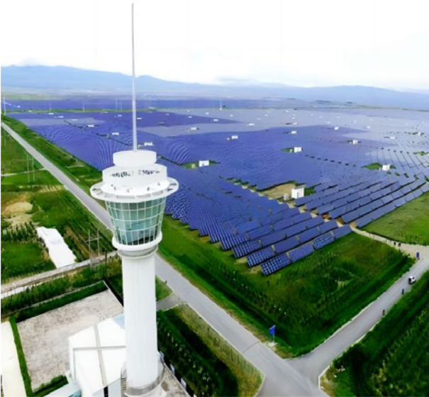
..... Figure 5-16 | Longyangxia hydro-solar hybrid project
