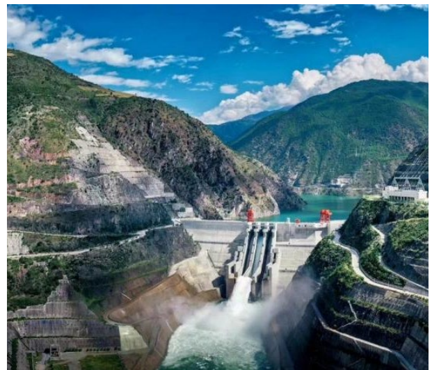
Figure 5-1 | Huangdeng hydropower project
