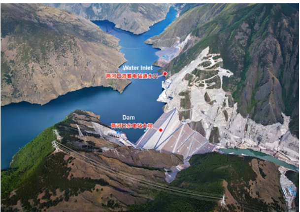
Figure 5-15 | Lianghekou hybrid pumped storage power station on the Yalong River
